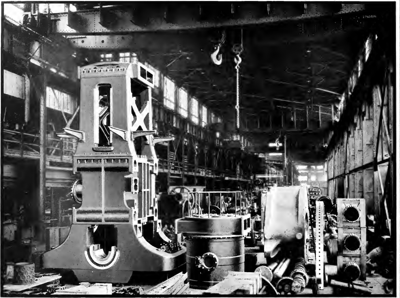
Vertical Long Crosshead Type Blowing Engine on Erecting Floor
